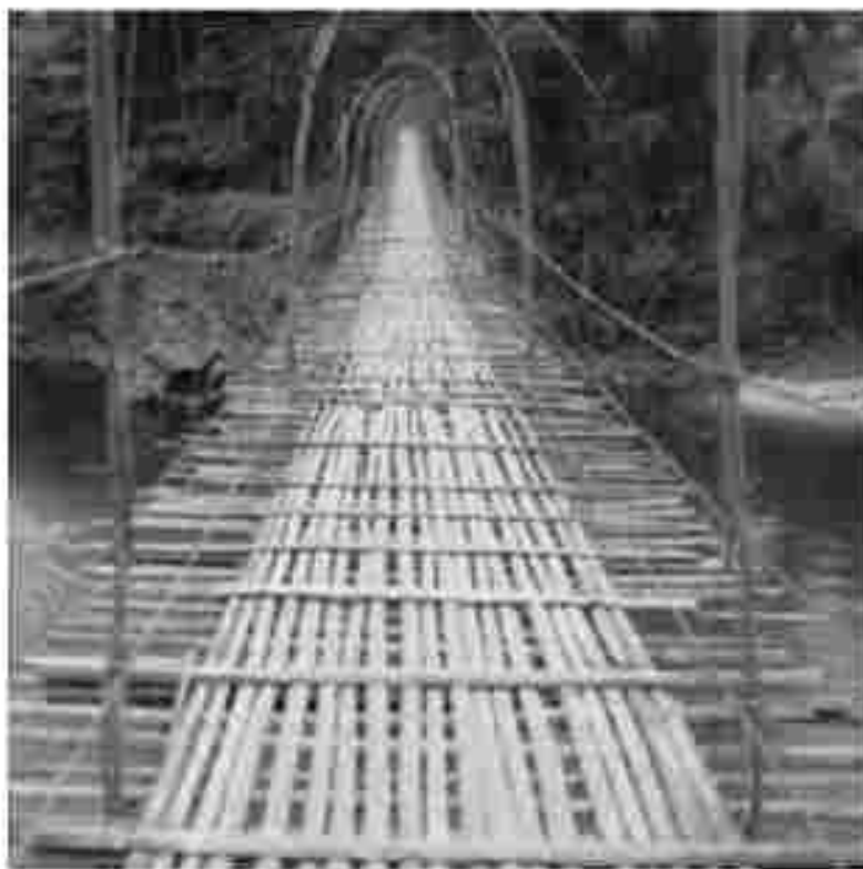
Cane and bamboo suspension bridge over a torrential river in Apong, Arunachal Pradesh.
